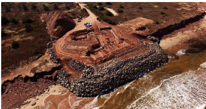
Point Deroche following Hurricane Fiona
